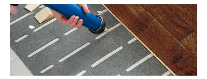
NAIL DOWN INSTALLATIONS – We do not recommend nailing only, there is a possibility that the nails may squeak as the floor expands or contracts. We therefore only recommend nailing if carried out in conjunction with a full stick down.
